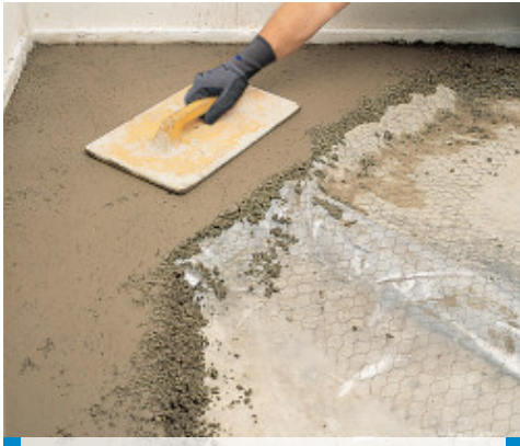
Covering pipes with Mapecem and reinforcement netting
