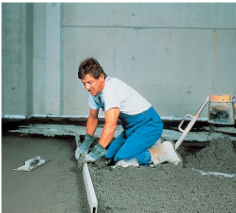
Using the straight-edge
