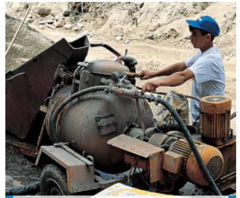
Mixing Mapecem with an automatic pumping unit
