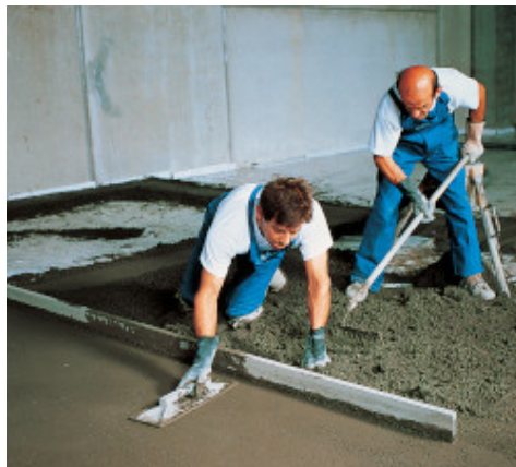
Tamping the Mapecem screed
