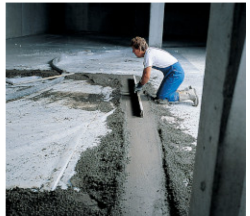
Preparing a levelling strip
