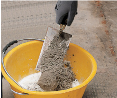
Mixing Mapecem with Planicrete SP to make a bonding slurry
